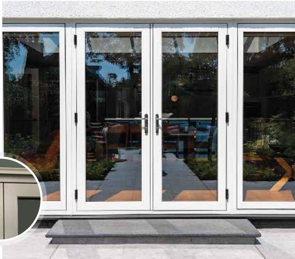
To achieve the most authentic finish for French doors that feature side panels, we intentionally use a deeper section to both the head and the cill. The resulting effect is that glass heights are all equal, providing a much more consistent sightline. Overall, they have the same appearance as traditional timber doors.
